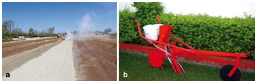
Fig. 5.2 a Spreading lime prior to ploughing; b animal-drawn seeder fitted with lime hopper
